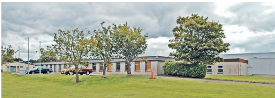
Tillotson's facility at Tralee
